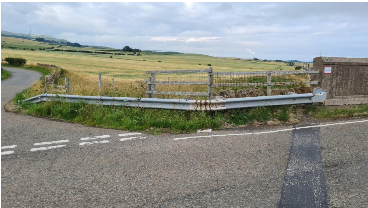
Photo 6 – Armco Barrier to be removed
