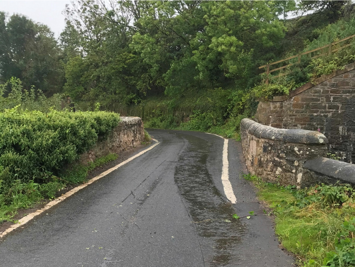
Photo 1 – Water crossing to be structurally assessed for HGV
