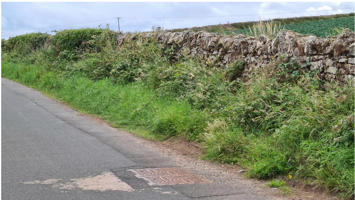
Photo 14 – manhole cover to be checked for loading capacity
