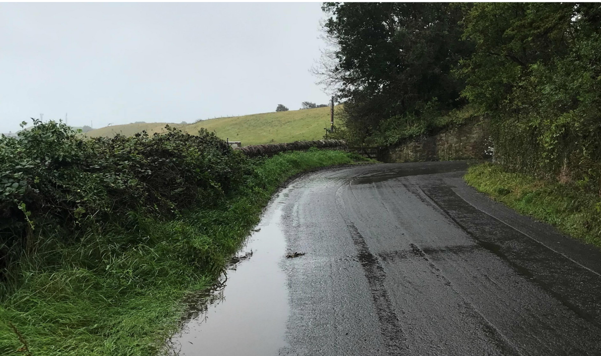
Photo 2 – Stone wall to be removed for vehicle over-run
