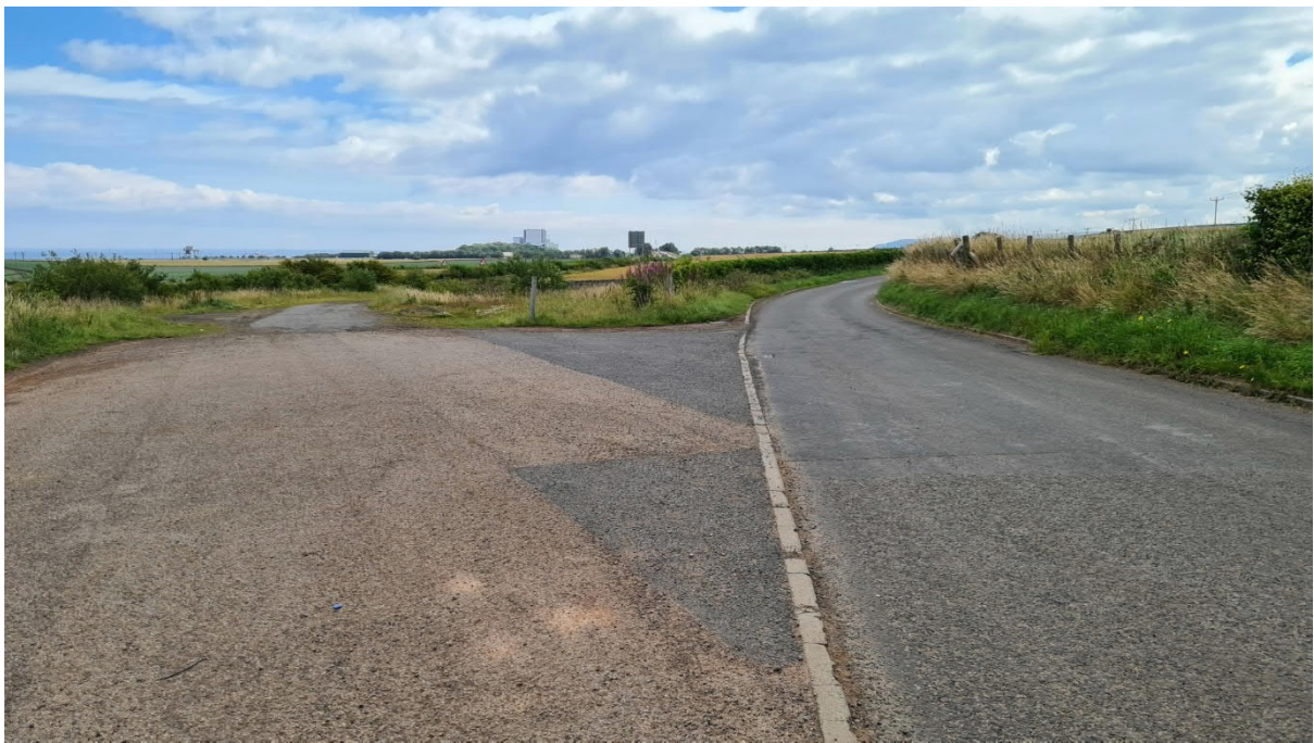
Photo 8 – Bend at Chainage 400 Drawing 102
