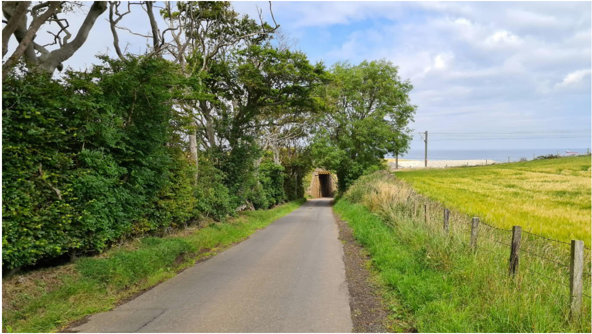
Photo 9 – View down toward railway bridge/ x-road location. Note steep embankment on RHS and mature trees LHS.
