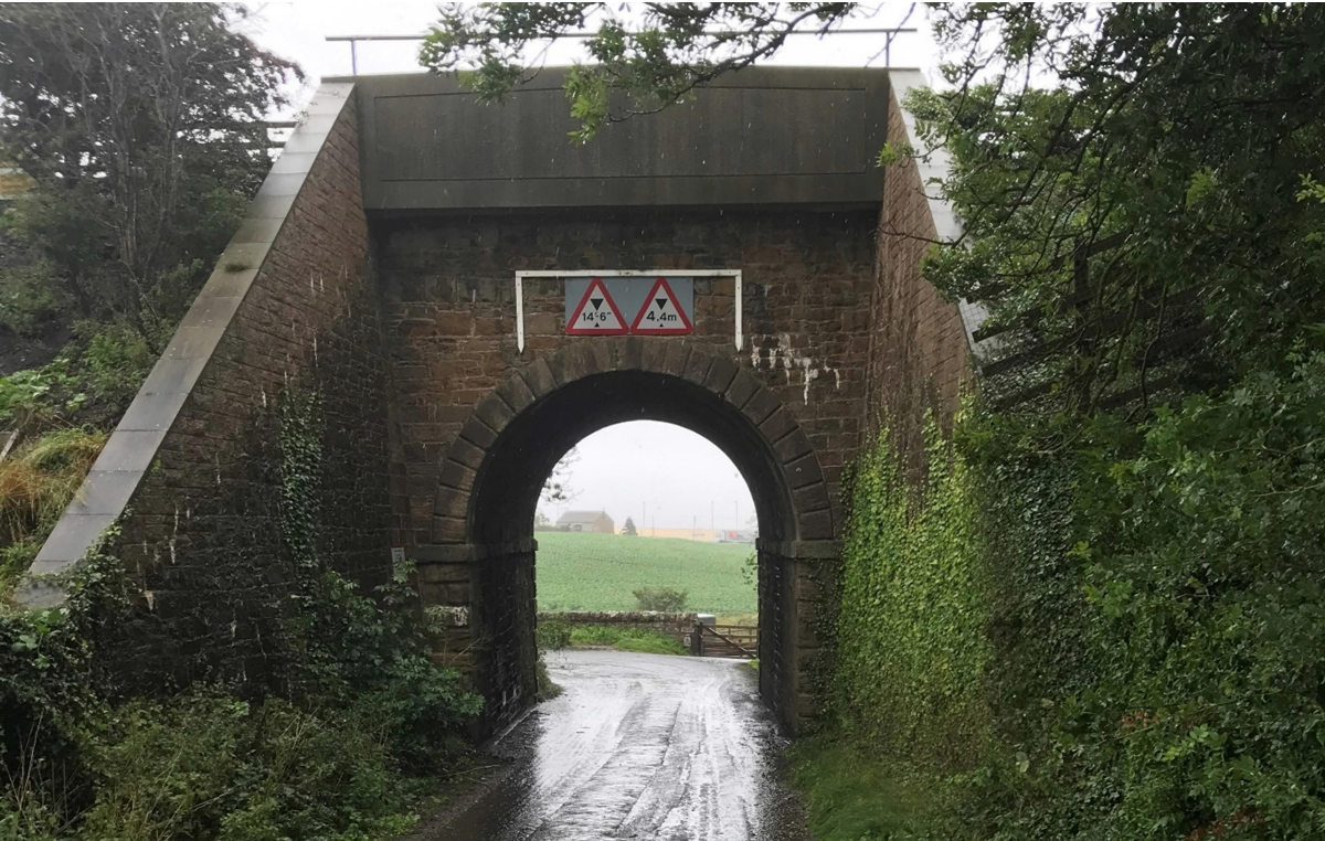
Photo 4 – Railway bridge crossing (looking back through towards stone wall)
