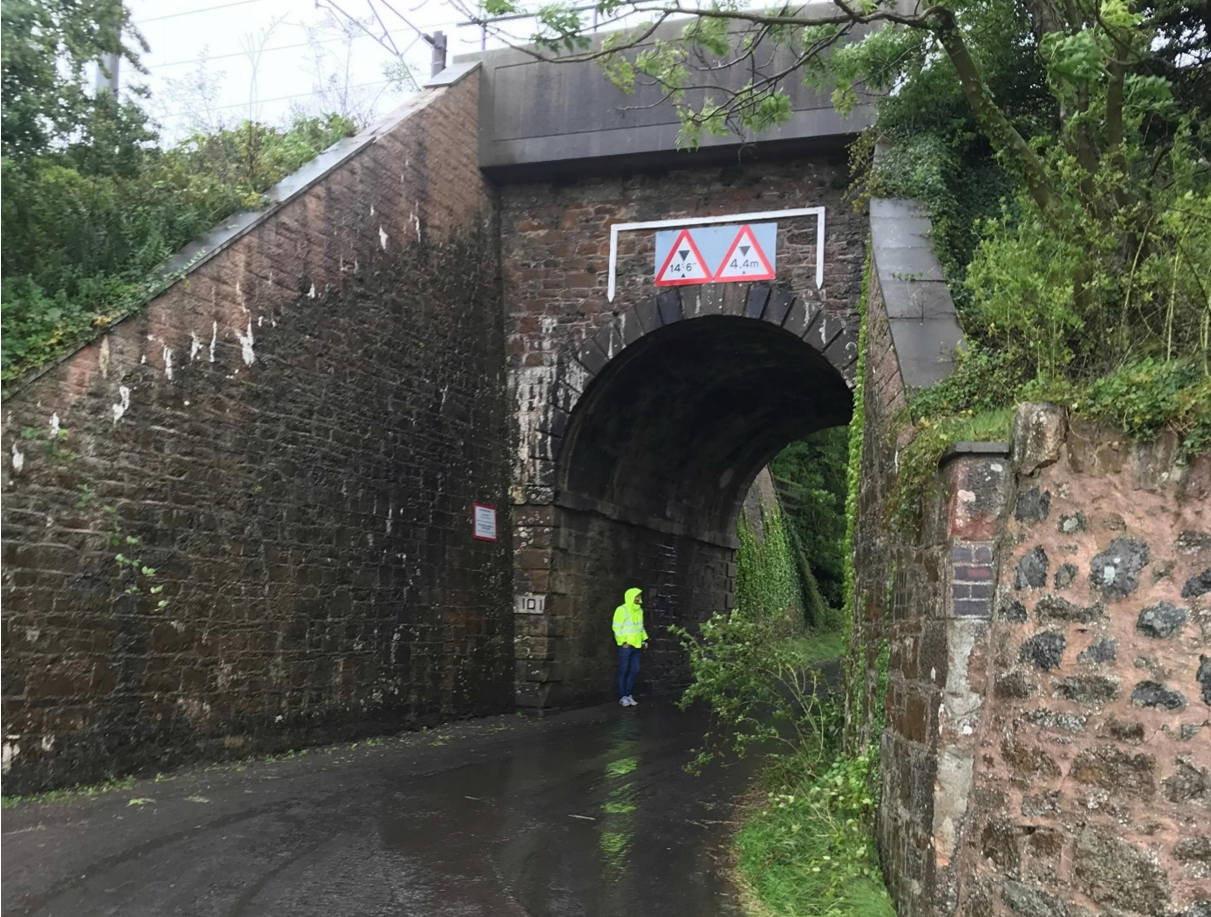
Photo 3 – Railway bridge crossing
