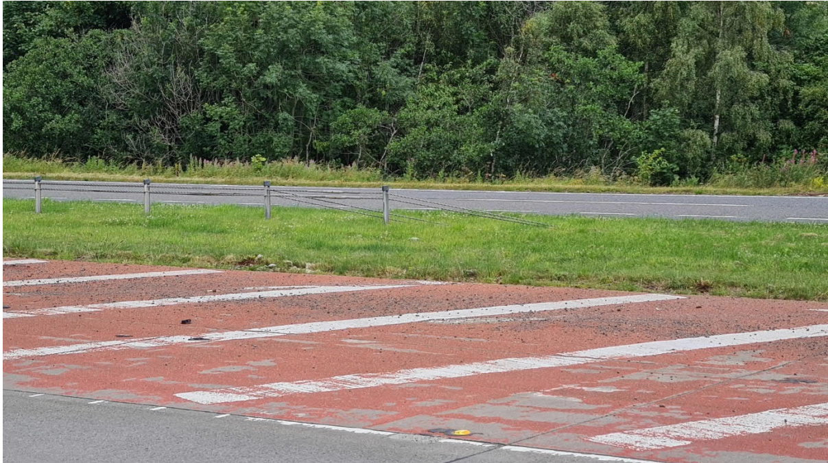
Photo 1 – Barrier to be removed at A1 Junction
