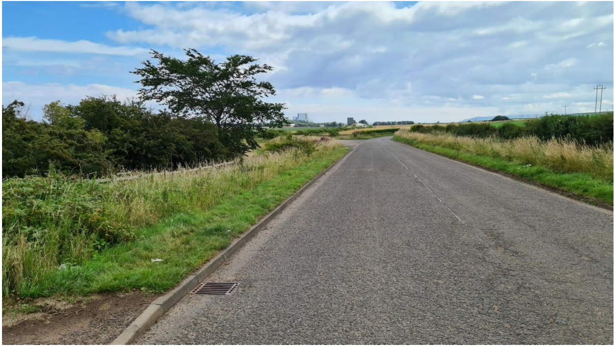
Photo 7 – View up access route after left turn
