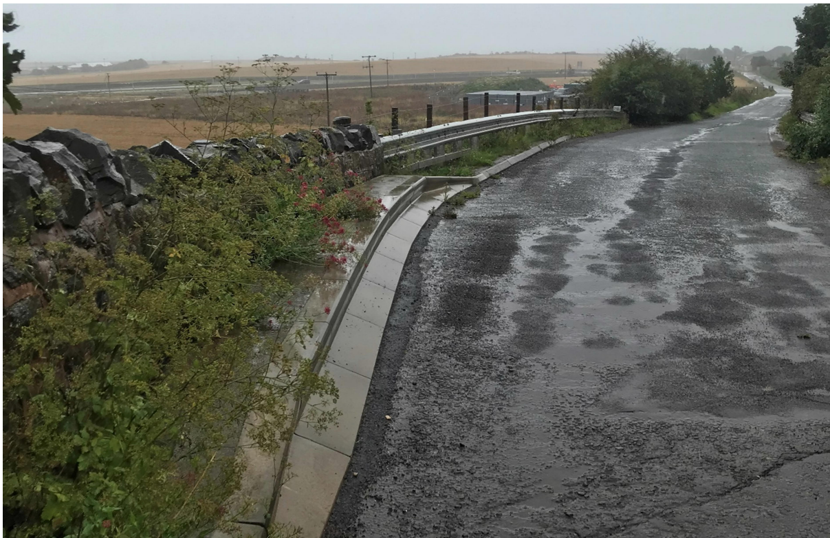
Photo 2 – Approach to Railway bridge (looking from bridge)
