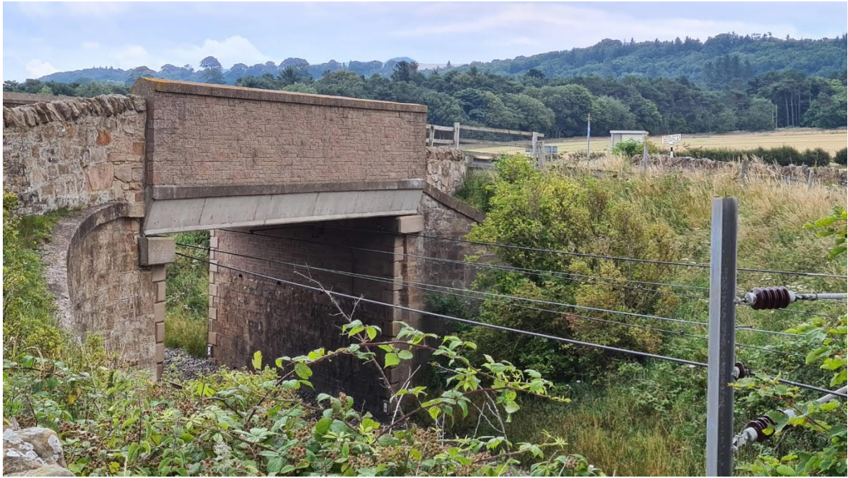
Photo 5 – Railway bridge parapet to be removed
