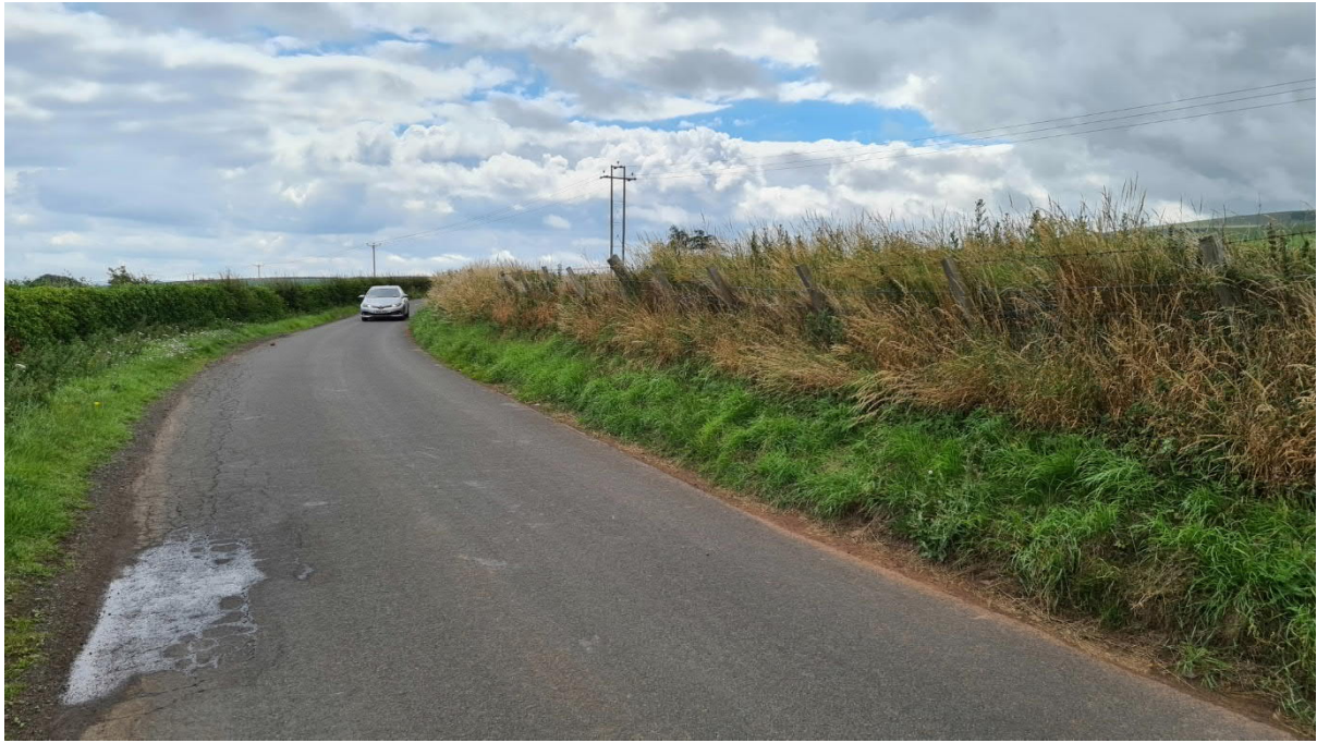
Photo 9 – Fenceline/Foliage to be removed
