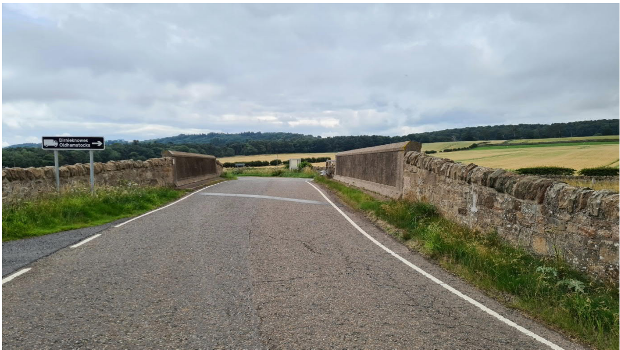
Photo 4 – Railway bridge for structural assesment
