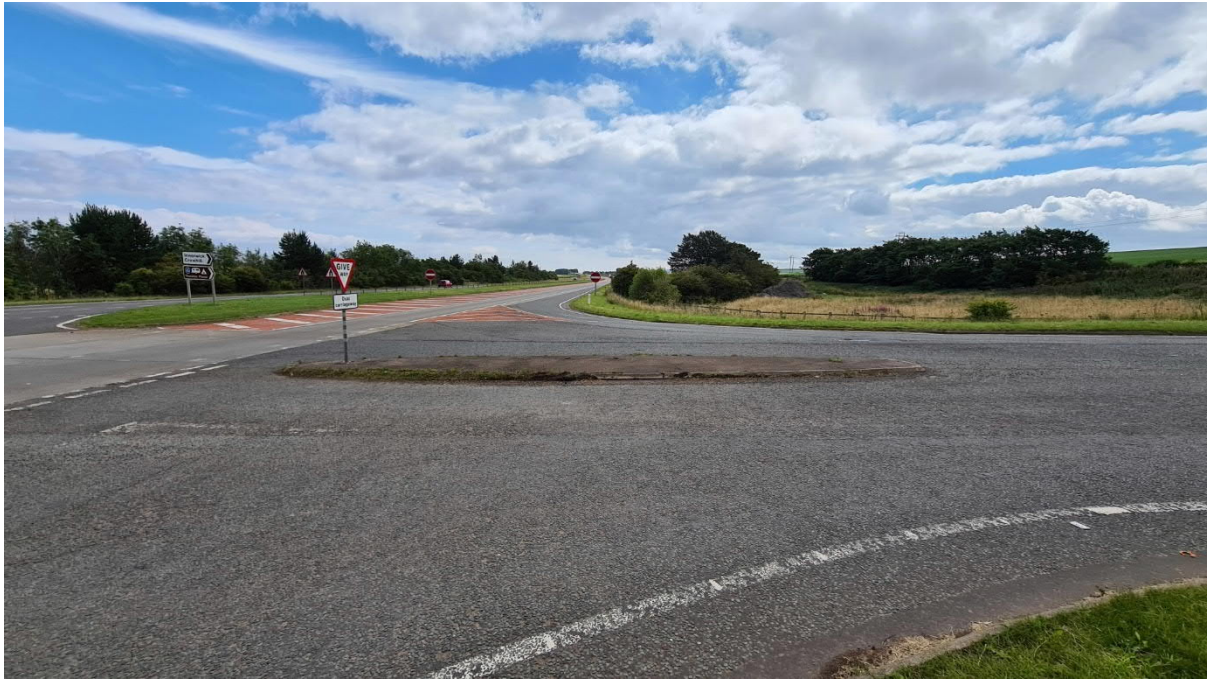
Photo 3 – Central island/road sign to be removed.
