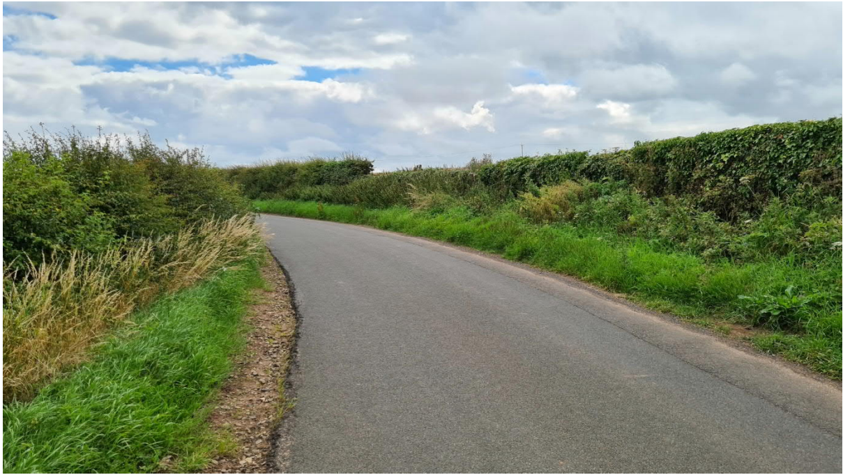
Photo 15 – Foliage/fenceline to be removed to accommodate overswing
