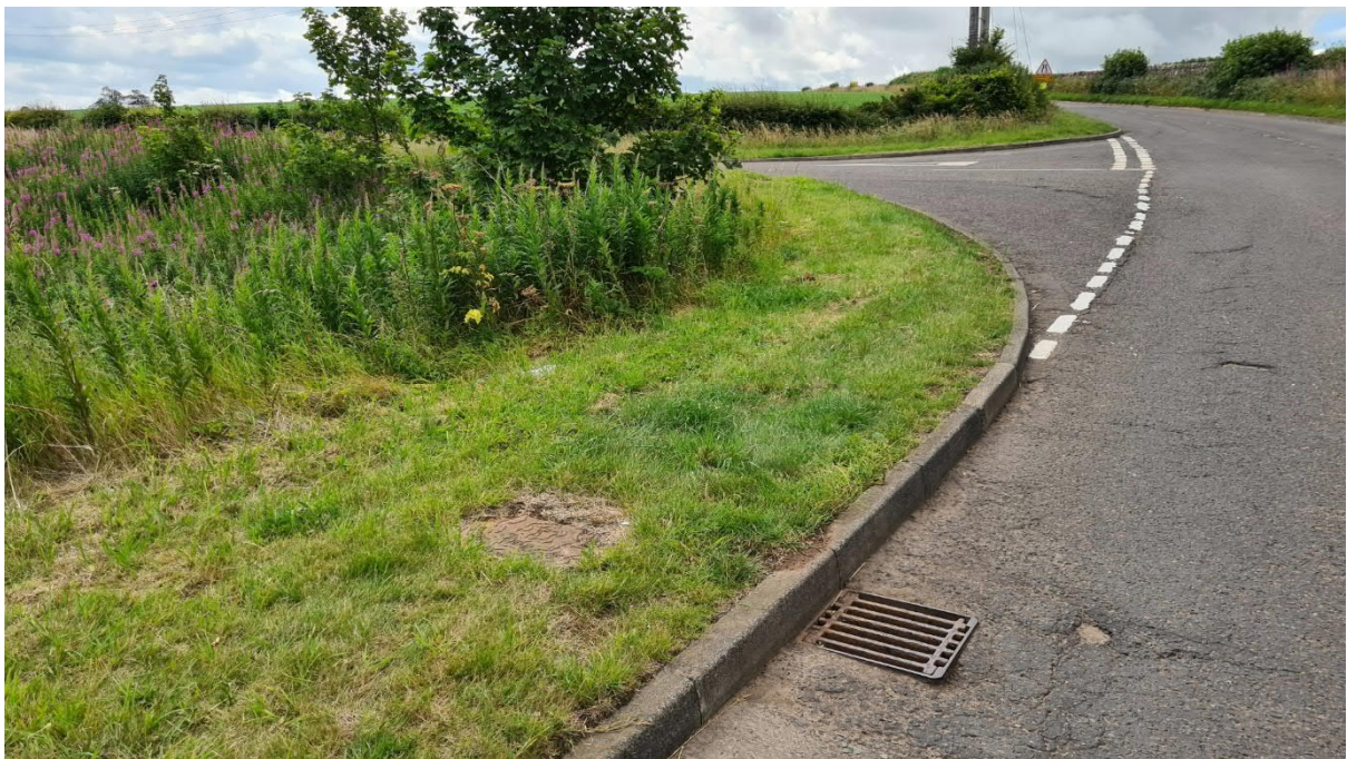
Photo 6 – Manhole/drain cover to be inspected for load capacity
