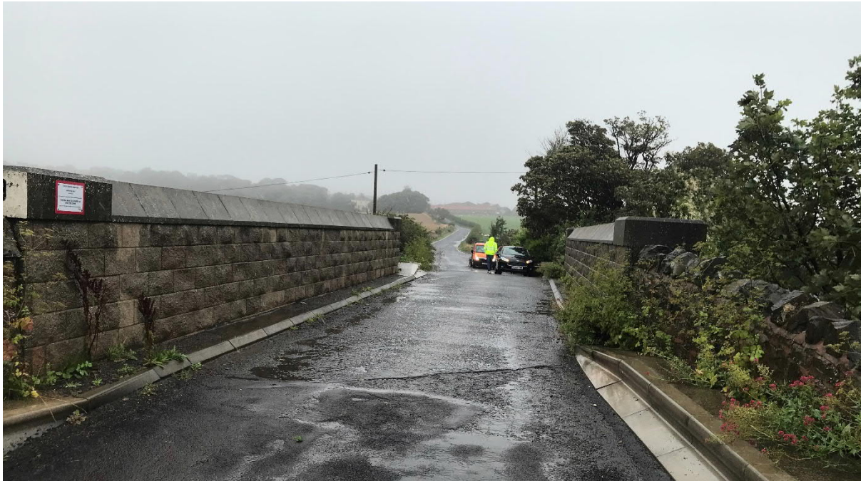
Photo 1 – Railway bridge to be structurally assessed for HGV
