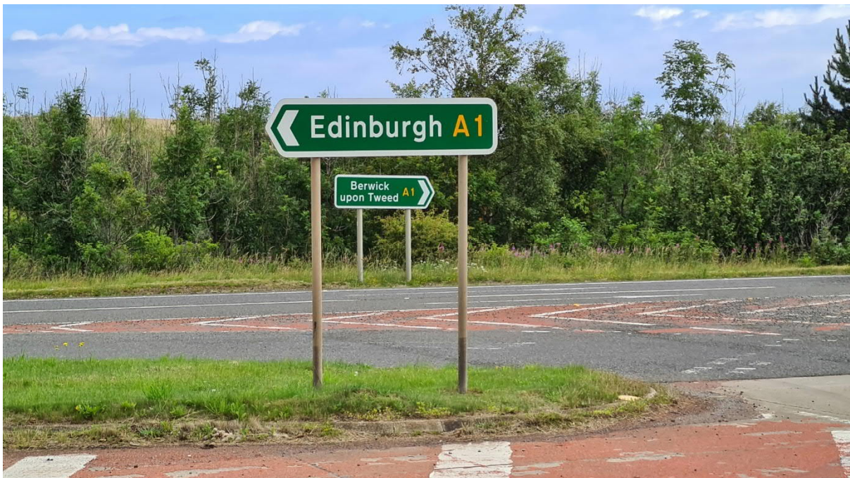
Photo 2 – Signpost to be removed/central reservation overrun area
